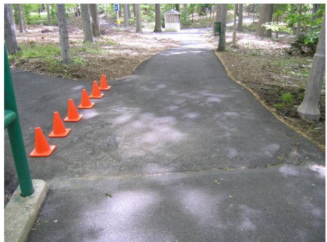
Figure 3: Campus Path with Orange Cones
