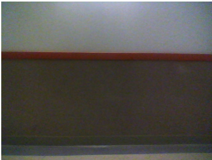
Image of the wall
