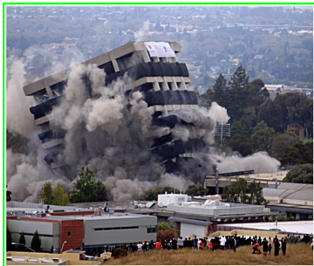
Anybody Could Have Tripped Over That Wire!
